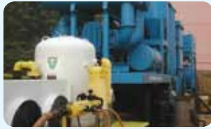
Dual D54 dryers (left) are used at a landfill to remove moisture from low pressure methane. A D36 dryer (right) is used to remove moisture from compressed air on a steel grit recycling trailer.
